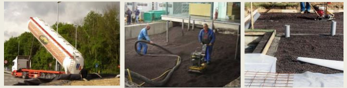
Figure 3: Blowing with vibrating plate levelling-compaction installation
