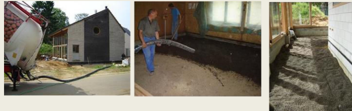
Figure 4: Blowing with manual levelling installation
